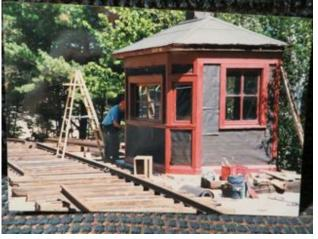
The scale is about sixty feet in length and easily handles a fifty-foot car. The Weigh-master would stamp the weight ticket and affix a weight ticket to the waybill and insert the tare wt of the empty car.
