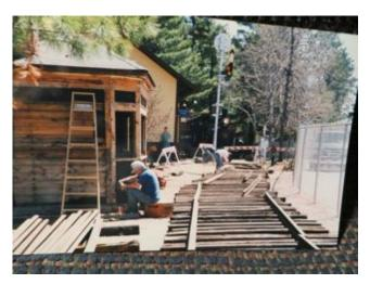
To the right, Norman is putting the finishing touch on a coat of paint. The walls are covered with tar-paper to help insulate the interior from the elements.
